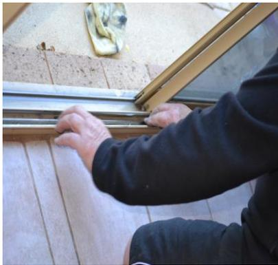
**#4. No screws are required to fit a *Miracle* Cover Track and no worry about galvanic corrosion problems.**
