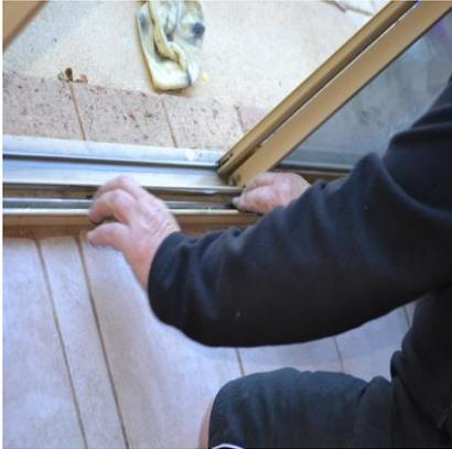
Step 4. Push cover track over existing track and press down to squeeze out resin filler. Do not worry about cleaning up any excess resin filler at this stage. Very important to have track seated before resin filler begins to gel.
