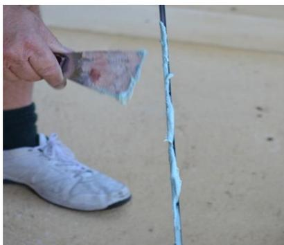
Step 3. Using a flat blade, fill the *Miracle* Stainless Steel track with the mixed polyester product. Use the flat blade to remove excess from back of track.
