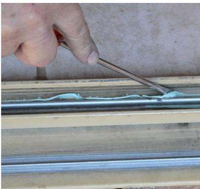
Step 5. Once resin filler has gel set, use a flat screwdriver blade to run along both sides to clean out excess filler product. This is a quick and clean process. Use a vacuum to suck out loose material and job is done.
