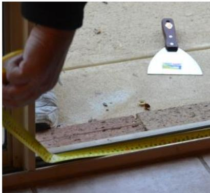
Step 1. Measure and cut track to length then test fit. Clean track to be free from dirt, oils etc.
